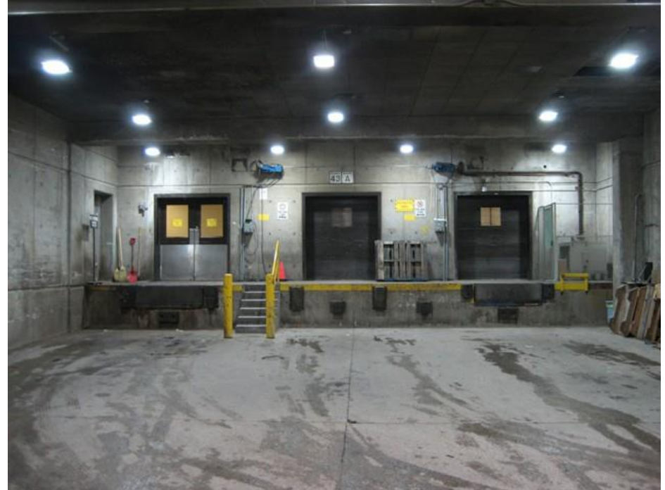
Loading dock location & height. No roll up ramp. Yet dock leveler for loading and unloading.
